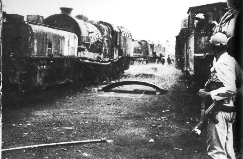
A graveyard of steam engines at Munhango in Angola on the Benguela Railway
